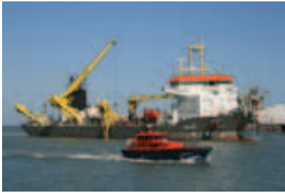
Dredging in the Inner Harbour.
