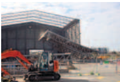
Demolition of the large shed on Berth 12 began in April 2011.
