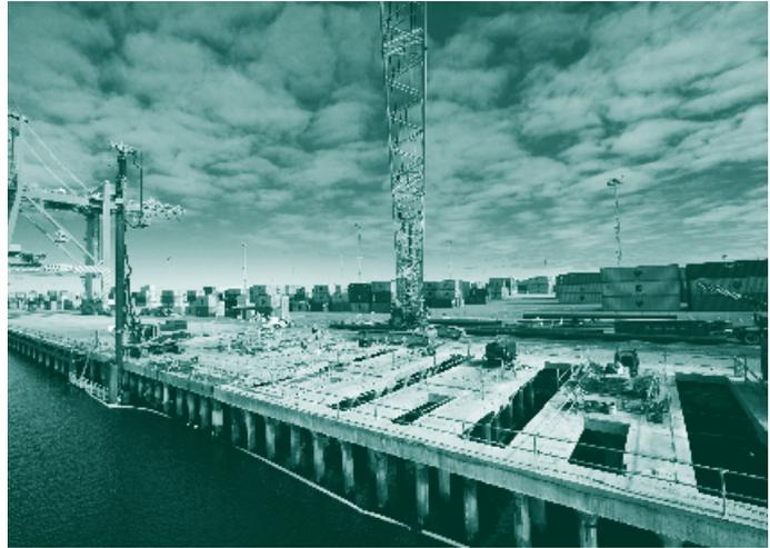
Berth 10 is being replaced with a stronger structure to allow it to be used for container ships.
