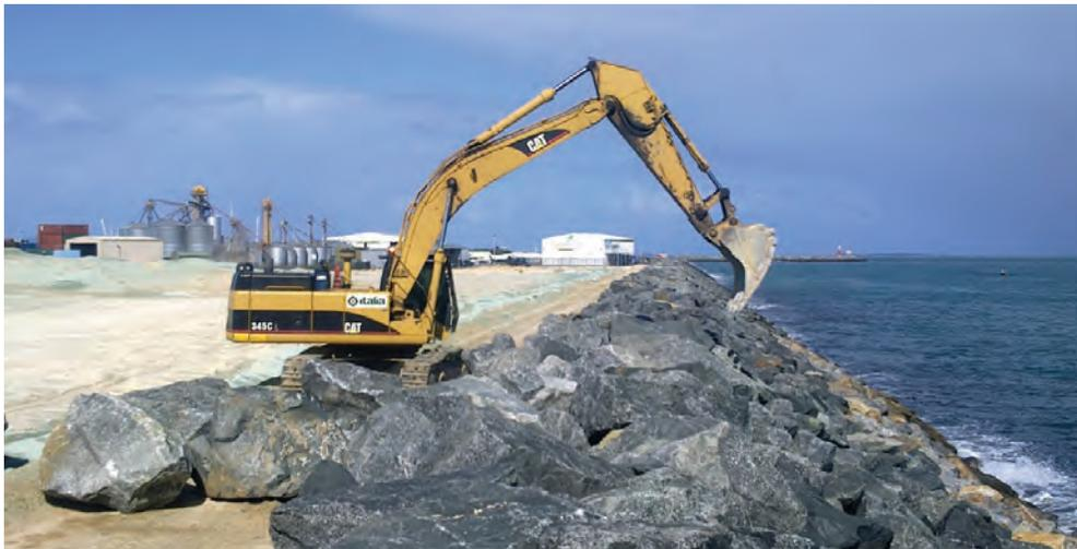
Armour rock repair to damaged seawall at Rous Head
