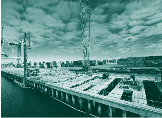
Berth 10 is being replaced with a stronger structure to allow it to be used for container ships.
