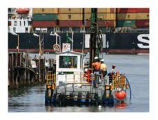
Core sampling for geotechnical analysis at the Fremantle Rail Bridge.
