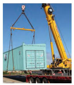
This 26-tonne electrical substation, is one of nine fitted out at Slip Street, Victoria Quay as part of the upgrade of the high-voltage electrical network on North Quay.
