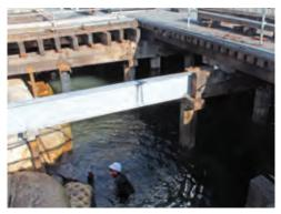
Wharf repairs at O'Connor Landing on Victoria Quay involved removal and replacement of damaged deck beams and installation of a new steel support.
