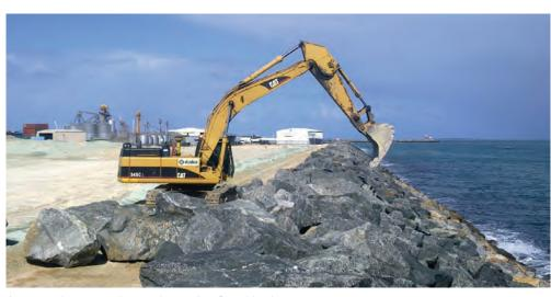
Armour rock repair to damaged seawall at Rous Head
