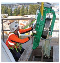
A new administration building lift motor being manoeuvred into place
