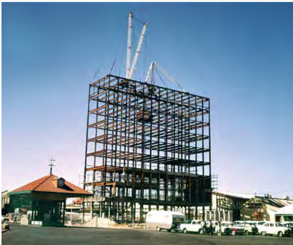
The steel frame of the building was completed in early 1963.
